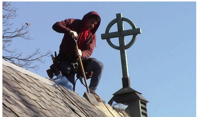
Workers expertly removed and replaced the church’s original slate roof.
